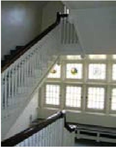
**Windows:** Replace broken window in kind. Some windows have experienced condensation damage due to the exterior storm windows. Replace third floor windows in kind as required.
