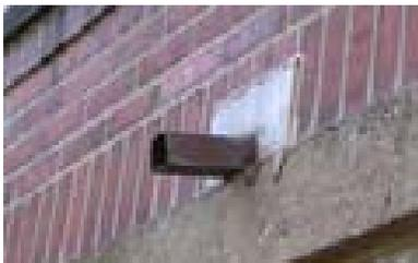
**Terrace Rain Leader:** Remove caulk and aluminum flashing. Restore to original opening size and design using copper flashing.
