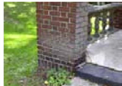
**Site Work:** At the front terrace, replace downspout scuppers to match the original design. Current scuppers do not extend far enough from the building; moisture is staining and damaging adjacent masonry.
