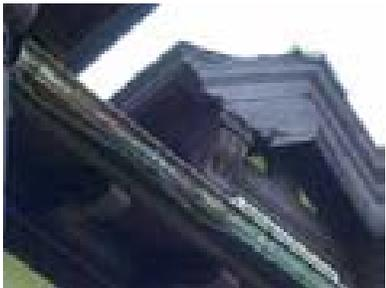
Deteriorated bargeboard trim and copper gutters on Mellon House.
