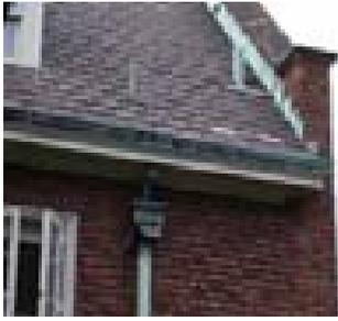
Parapets are a common location for flashing failure and masonry deterioration. This original, ornate, copper splash box at Rea House is in need of repair.
