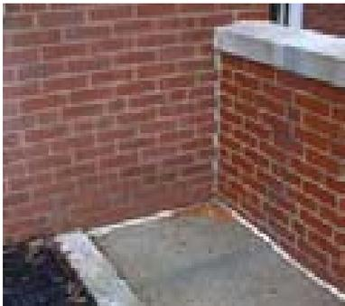
**Gutters:** Clean and repair as required. Replace in kind where required. Concrete at window wells is eroding due to overflow from clogged gutters
