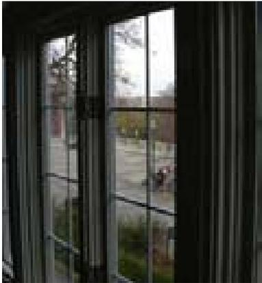
**Windows:** No windows are original, and many have been recently replaced. When windows are next replaced/upgraded, match the appearance, function and materials of the original window designs as closely as possible. Glass block and false-muntin replacement windows are not appropriate.
